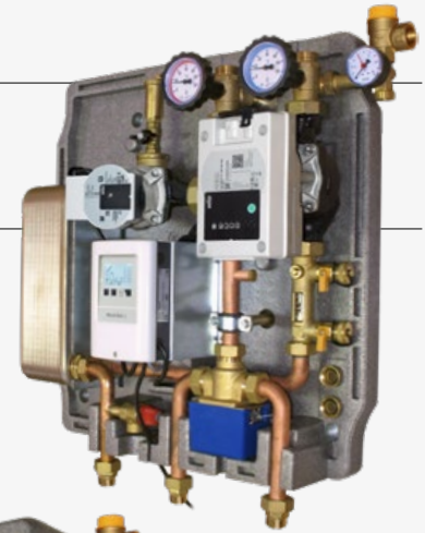
Pump unit assembled with optional ball valve kit
